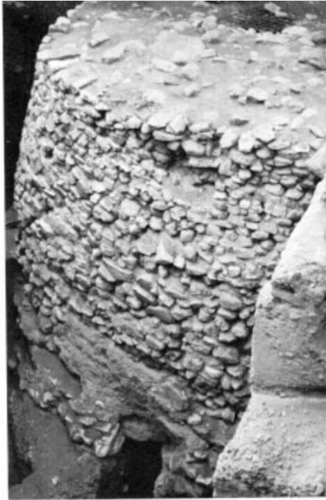
THE NEOLITHIC TOWER AT JERICHO. The steel grating at the top covers the opening to a narrow inner staircase that winds to the entrance at the bottom.
